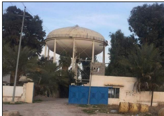
Figure 4. Elevated water storage tank at KCWTP
